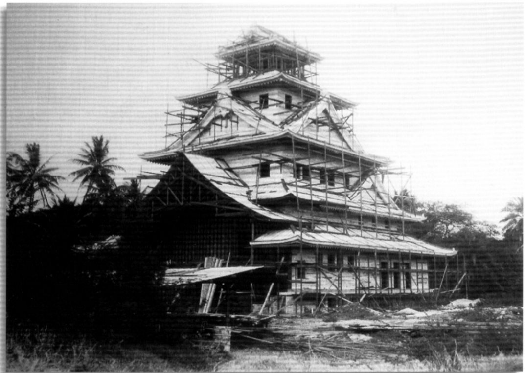
Construction begins; ca. 1931-1932
